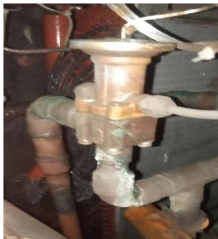
Fig 3. Expansion valve
