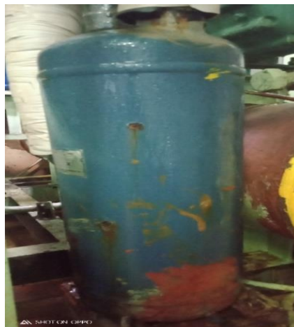
Fig 6. Oil Separator
