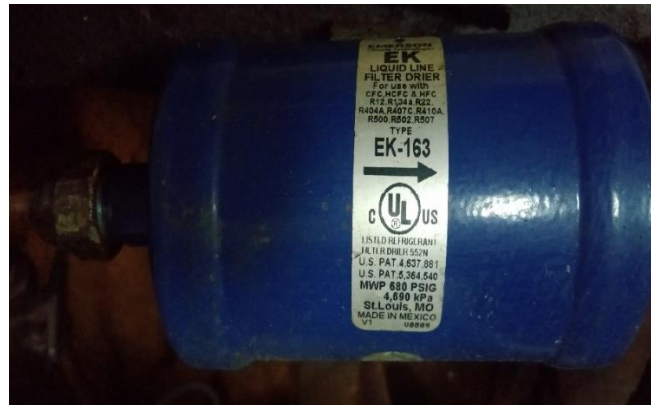
Fig 7. Filter dryer
