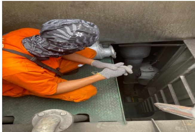
Fig 6. A/E II Silencer Leak Repair
