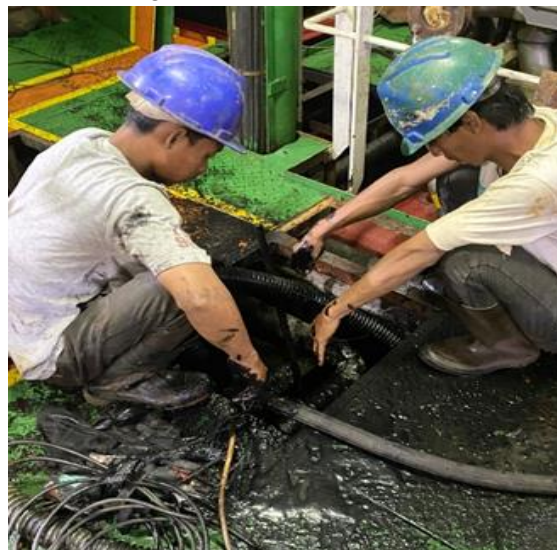
Fig 7. Cleaning the Ship's Bilge
