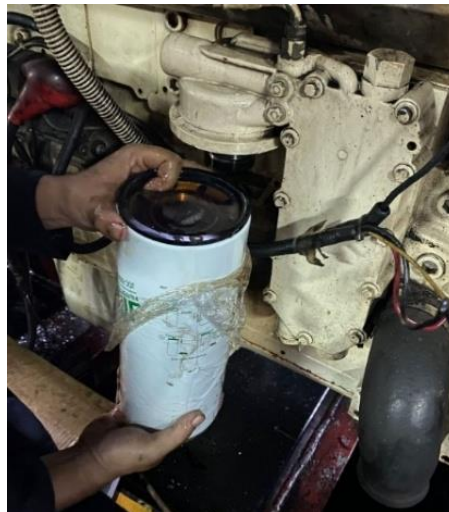
Fig 9. Replacing A/E Oil Filter III
