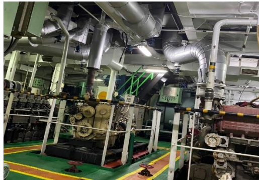
Fig 2. Engine room of KM Sabuk Nusantara 101
