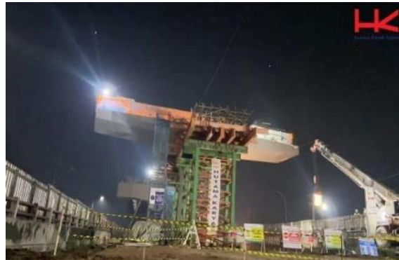
Fig 6. Application of Sosrobahu Technology (Source: Author Documentation, 2025)
