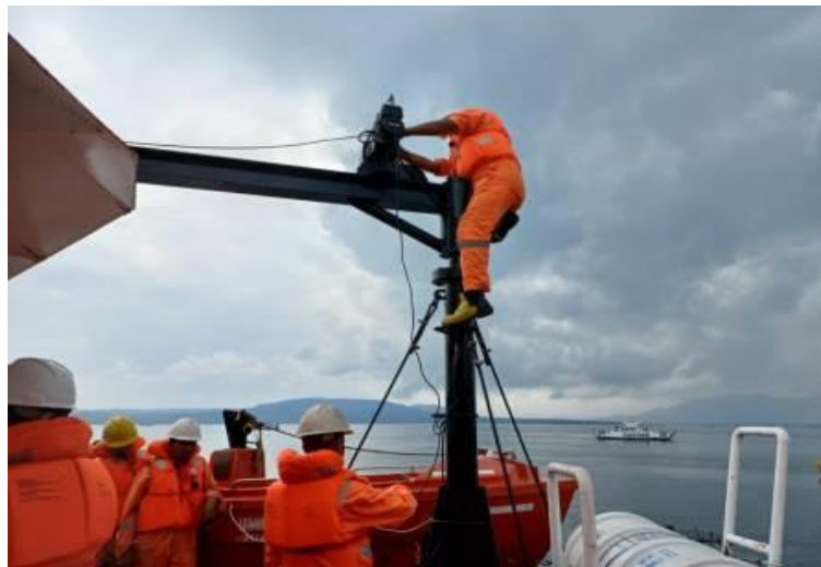
Fig 2. Inspection of Lifeboats on KMP Jambo VIII
