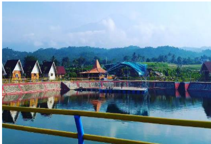
Fig 6. Banteran Dam has a water capacity of 21,000 m 3
